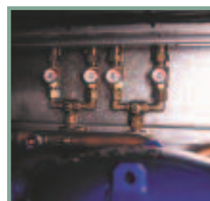
Dual pressure relief valve
